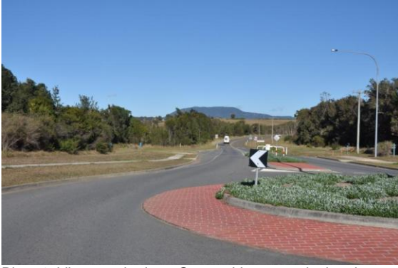
Plate 1: View south along Ocean drive towards the site.
