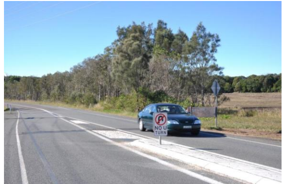
Plate 10: View east along Ocean Drive.
